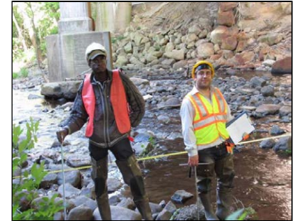
Student researchers, Dillion Collins and Abofazl Bayat, assess the pier foundations of a Northern Passaic County bridge .
